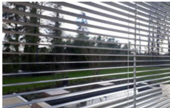
Conversely, the unimpeded heat input leads at days of extreme sun exposure to extreme stress for blind components. An essential role is played here by different expansion coefficients of individual components. The most heavily loaded are the
